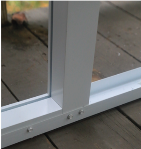
2x2 Mainframe in Bottom Uchannel
